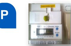
**Production meter** (or injection) shows the energy accumulation produced by your system since the installation of the meter.
