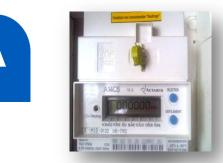
**Non-consumption meter** (or withdrawal, or consumption of auxiliaries) shows the energy accumulation consumed by your inverter mostly when your photovoltaic installation doesn't produce electricity.
